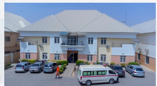
UMC Zhahir Hospital Kano, Nigeria
